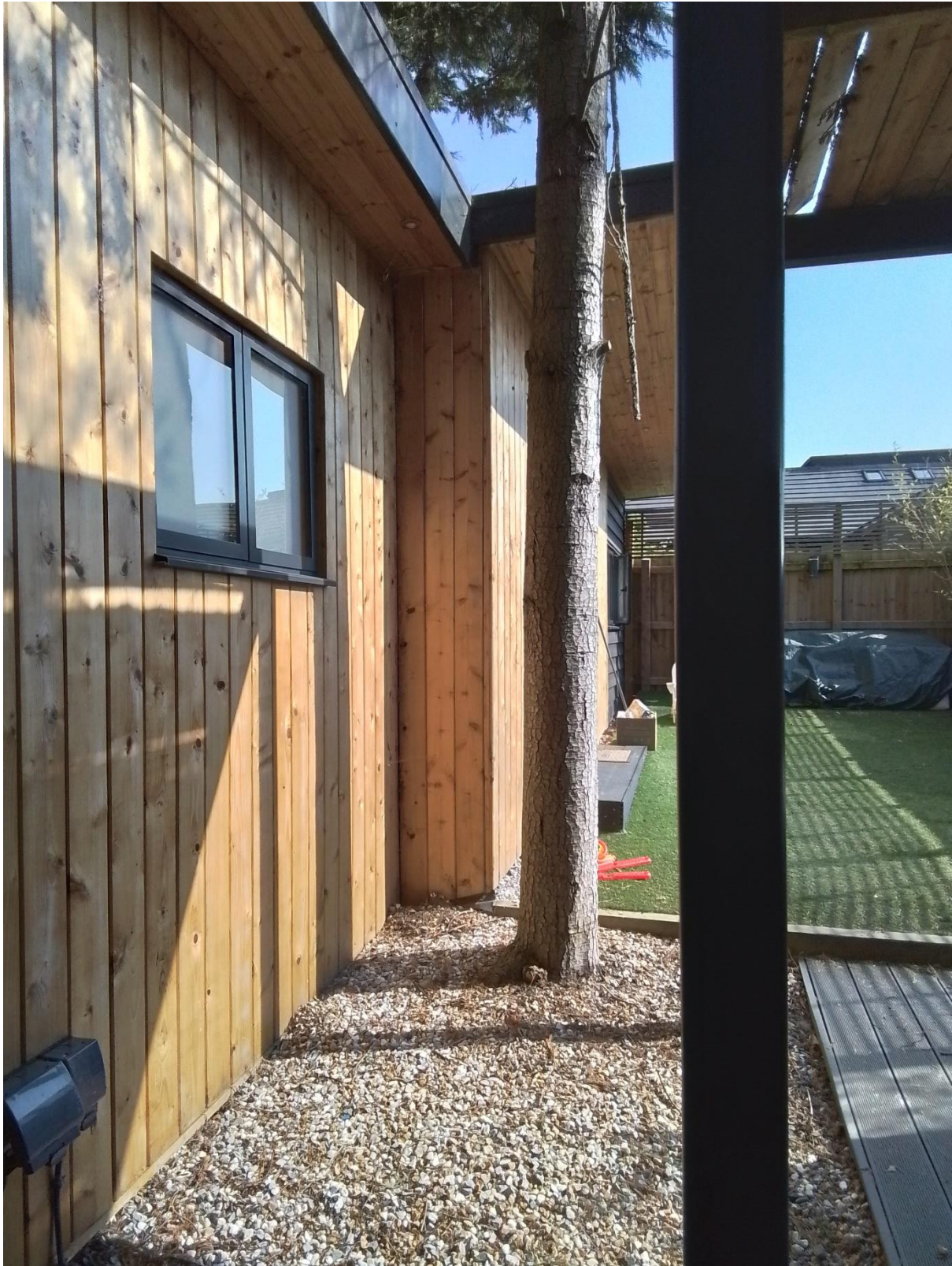
Front east elevation of Tree House
