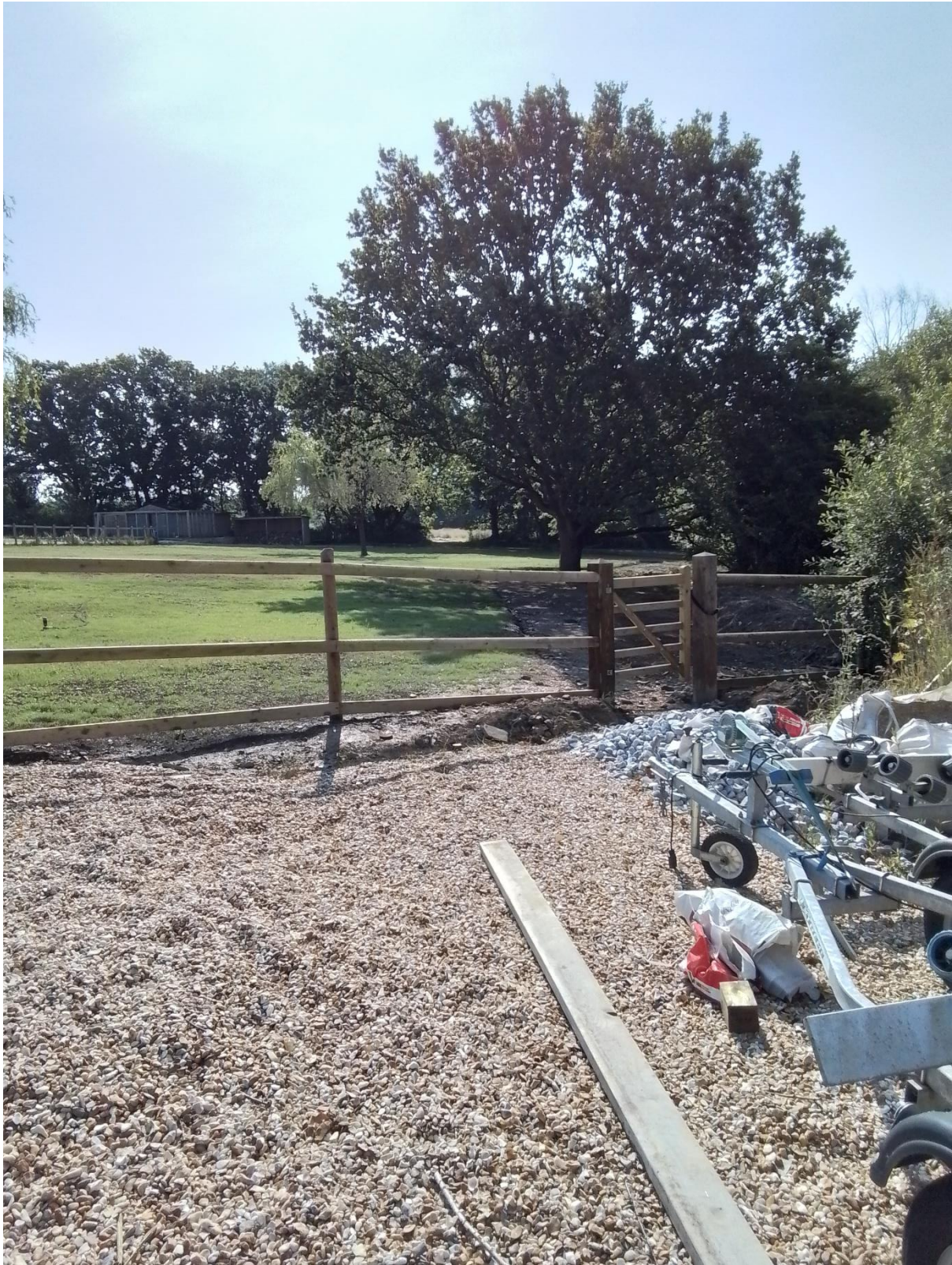
Garden of White Barn looking from Area 4
