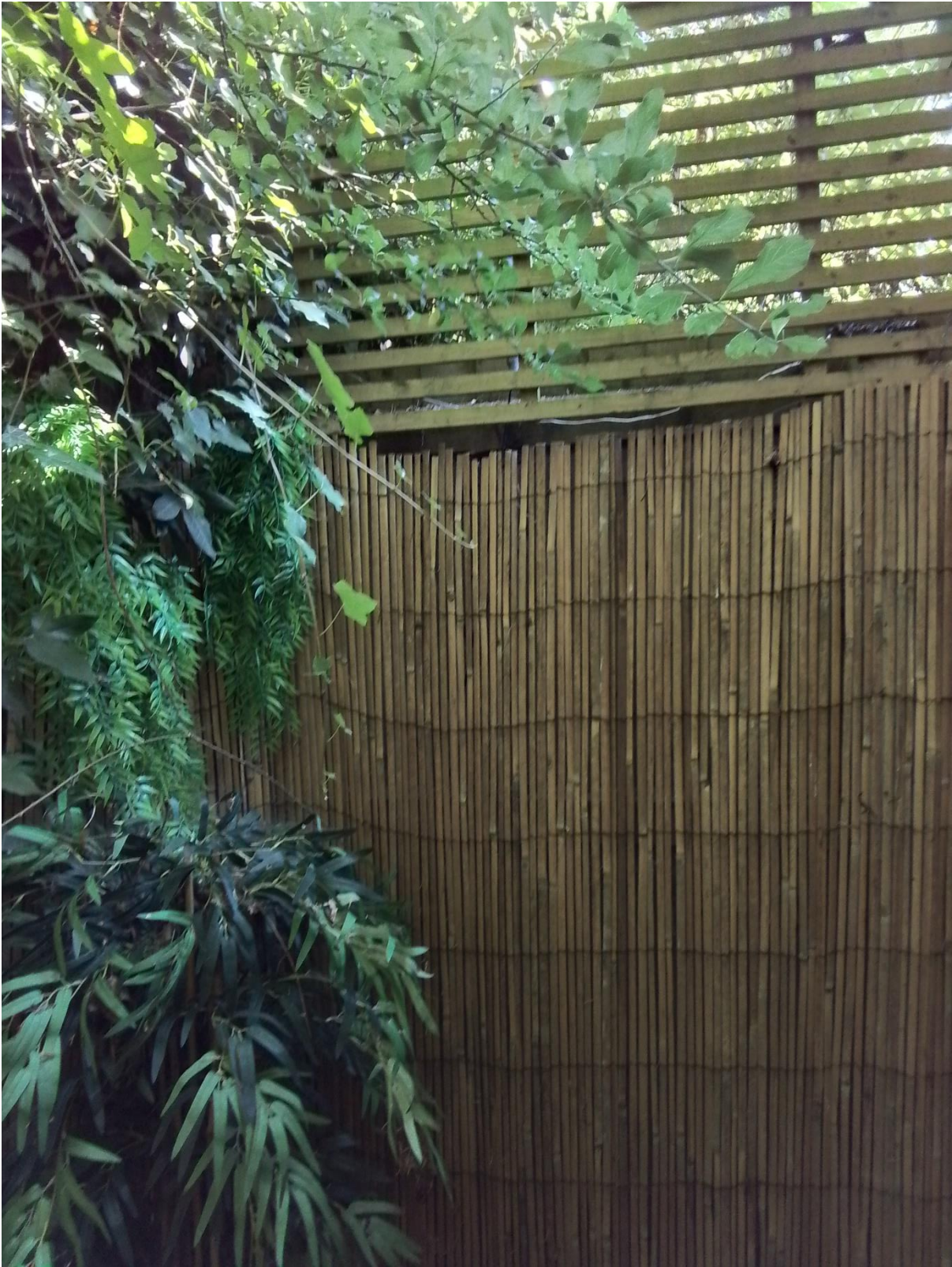
Fencing at rear of Tree House
